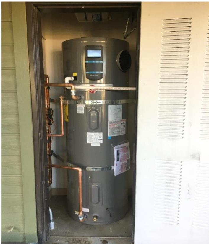
FIGURE 6: TYPICAL HPWH WATER HEATER CLOSET INSTALLATION
