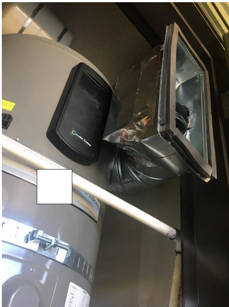
Figure 2: Gasketed Floor Register Position Relative to Open Door
